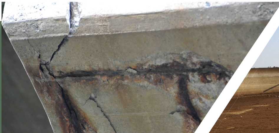
Catastrophic loss of concrete matrix integrity
