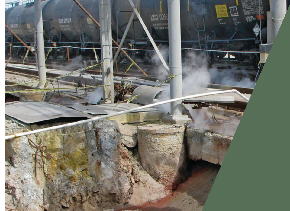
Symptoms of advanced concrete “cancer”
