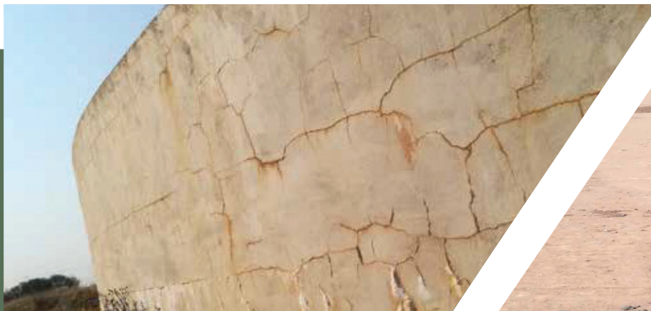
Indications of corrosion in steel-reinforced concrete matrix
